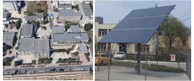
Fig. 1. View of LACARP PV system placement
