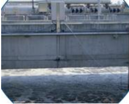
Figure 6 Measurements at several points of the aerator
